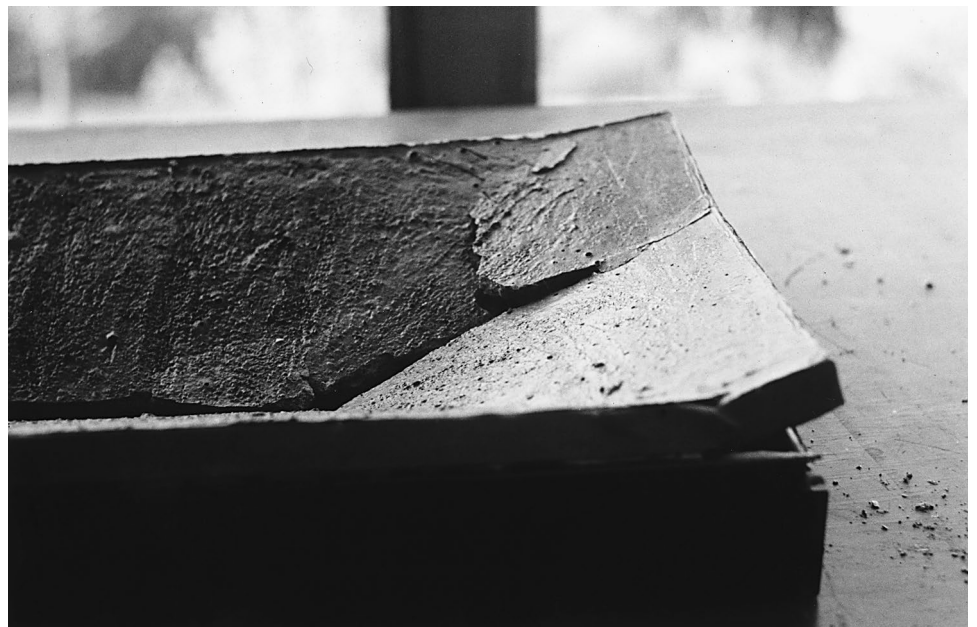
FIGURE 23.15 Development of corner levers in a simply supported, uniformly loaded slab. (Photograph by Arthur H. Nilson.)
