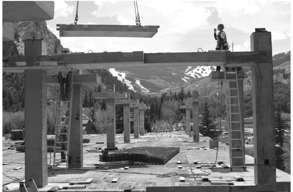
FIGURE 19.19 Precast slab element with precast columns, beams, and lateral framing. (Photograph by Charles W. Dolan.)
