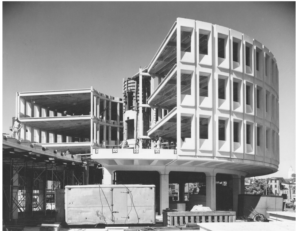
FIGURE 19.23 All precast administration building. ( Courtesy of Portland Cement Association. )
