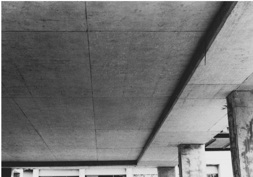
(b) Edge band at exterior column
