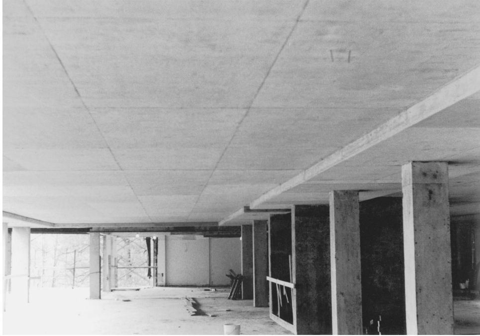
(a) Interior slab band
