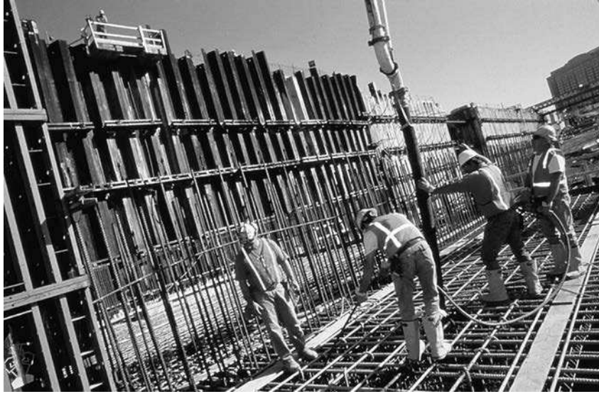
Colado del concreto, Big Dig, Boston, Massachusetts. (Steve Dunwell/Getty Images, Inc.)
