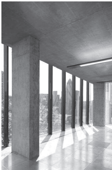
Losa plana sin vigas de borde. (Buckley Gray Yeoman, Fashion Street, Londres, 2010) (View Pictures/ UIG Getty Images, Inc.)
