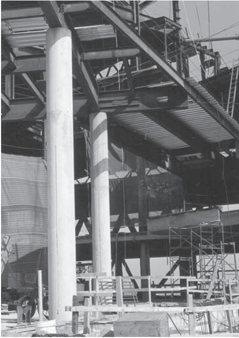
Columnas de concreto reforzado. (Cortesía de RSM Advertising, representando a Molded Fiber Glass Products Company.)
